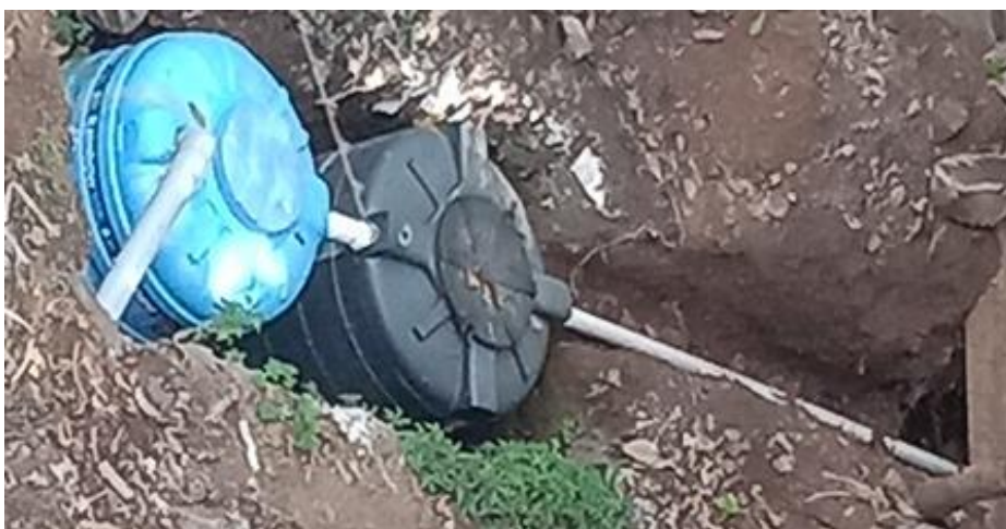
Laboratory wastewater neutralization set up
